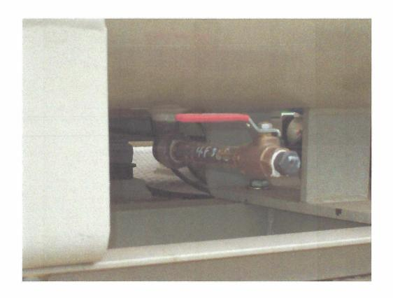
If an excessive amount of water is in the receiver tank is can get the air/oil separator filter wet and prevent it from filtering the oil from the air.
