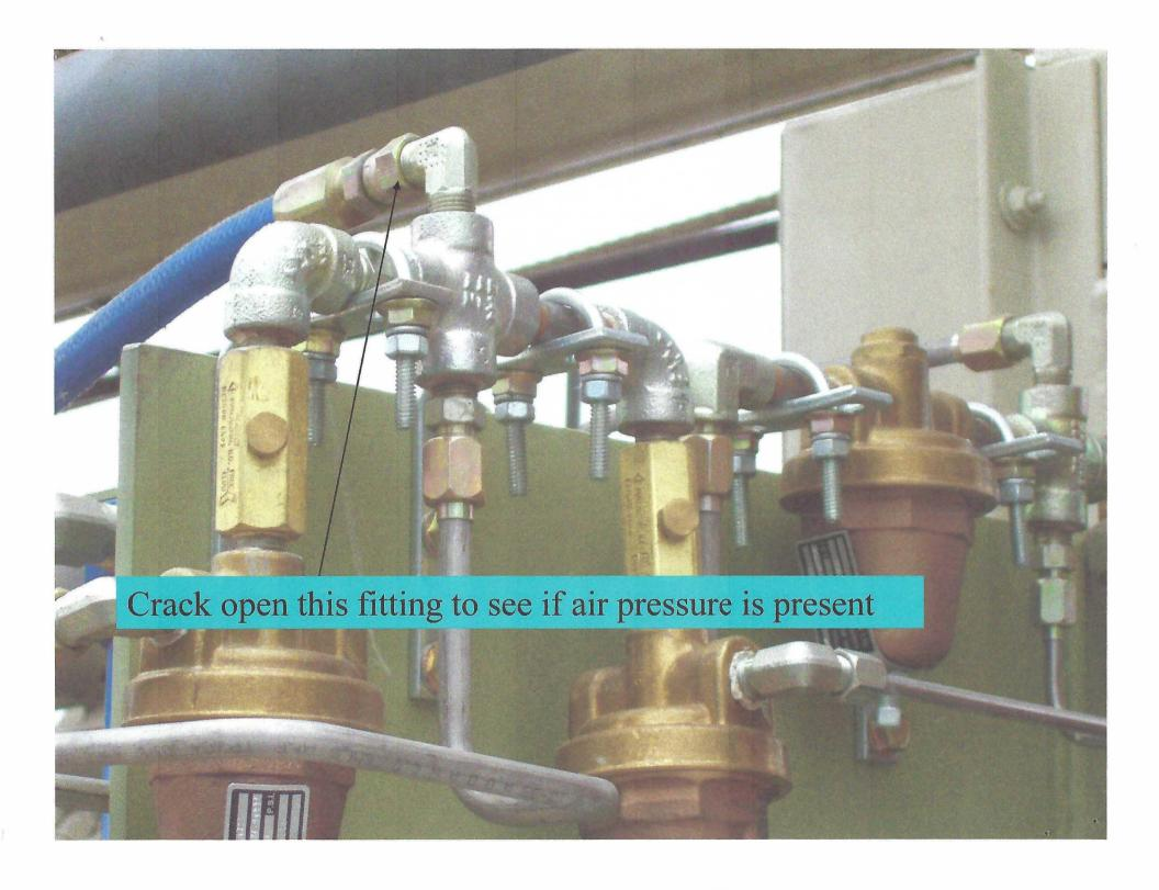
If air pressure is present, this means one of the regulators is opening and sending a signal to the inlet cylinder causing it to stay stroked closed. Many times the running blowdown valve will exhaust air at the same time. To determine which regulator is the problem, turn the highlow selector valve to the high position, if the air signal is lost then it is the low regulator, if the air signal remains then it is the high regulator.
